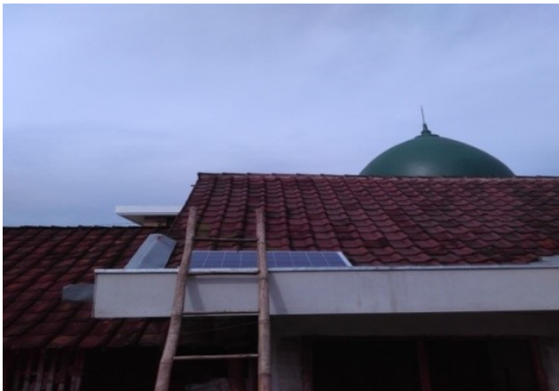
Picture 2. Solar Panel Installation.
