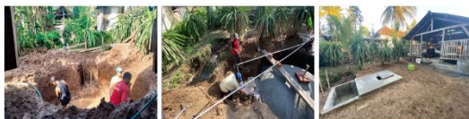
Figure 2. Digester Construction Process in the Field
